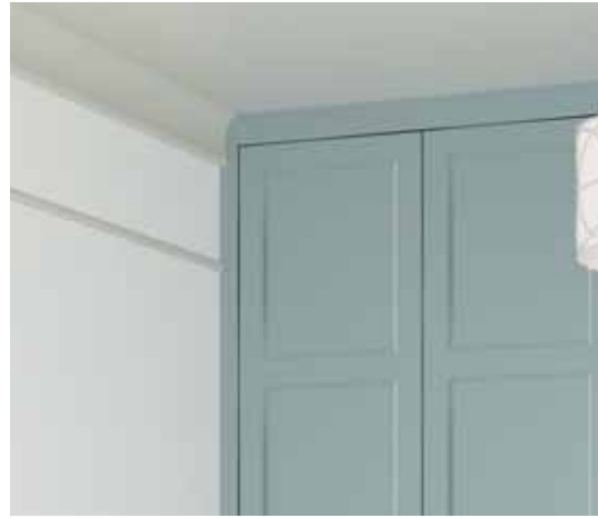
Plinth used as infill to ceiling
